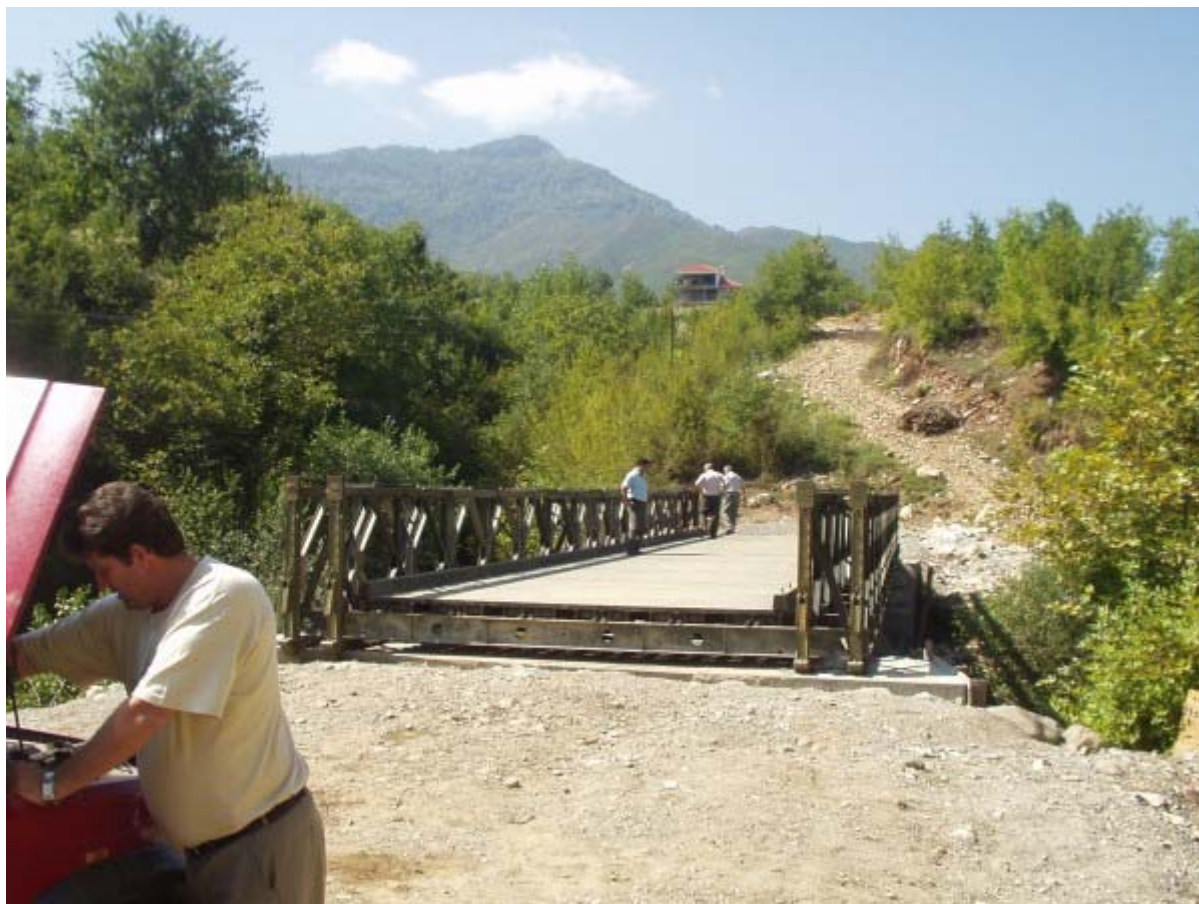
The Bailey bridge in Gurrë e Vogël. Photo: Bjoern Andersen
