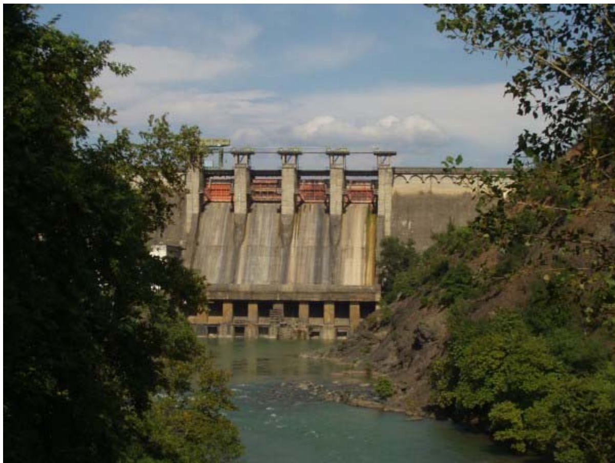
Mat Hydropower Station. Photo: Bjoern Andersen
